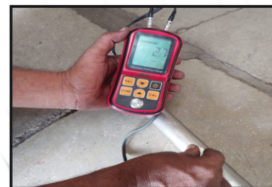
ULTRASONIC THICKNESS MEASUREMENT
